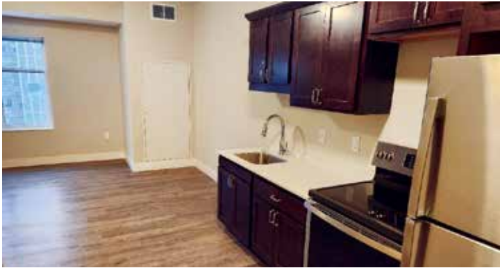
By January 2023, stainless steel appliances and classic dark cabinets had been installed in this apartment kitchen.
