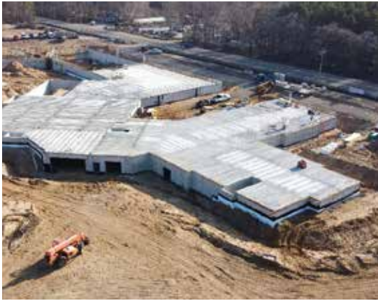
An aerial shot of the campus taken in early May after the site had been excavated and the footings and main level floor had been poured.
