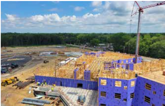
Much of June was spent framing and installing walls for the multilevel senior living building. By mid-July, work had begun on the roof parapet at the building's south end.
