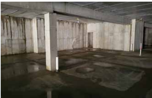
A view of the main building's basement after the concrete floor had been poured in late June. The basement will have underground parking spots for residents, along with a pet washing station, workshop, and production kitchen.
